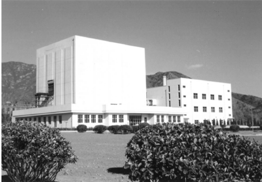
Figure 1 Chinese high temperature reactor (HTR-10)
